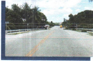
Local road projects
